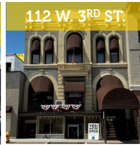
AMERICAN POWER SYSTEMS
